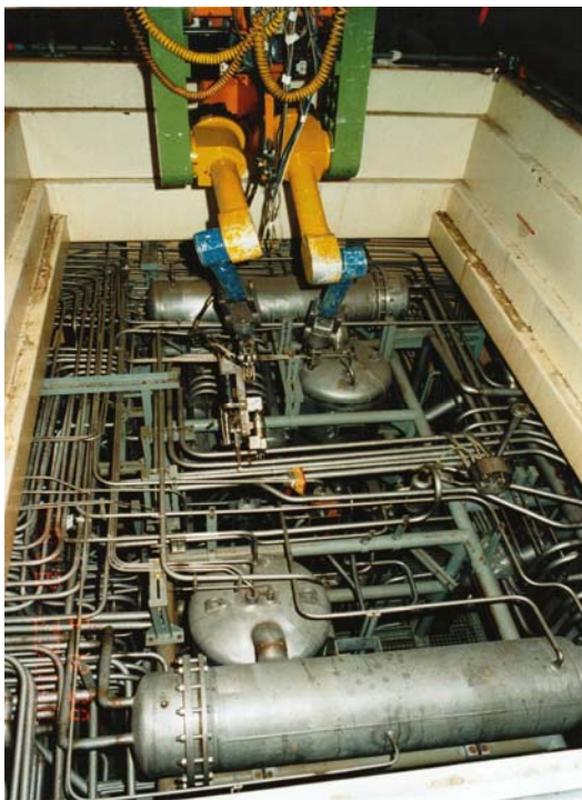
Figure 2: Remote dismantling of the HLLW evaporator cell
