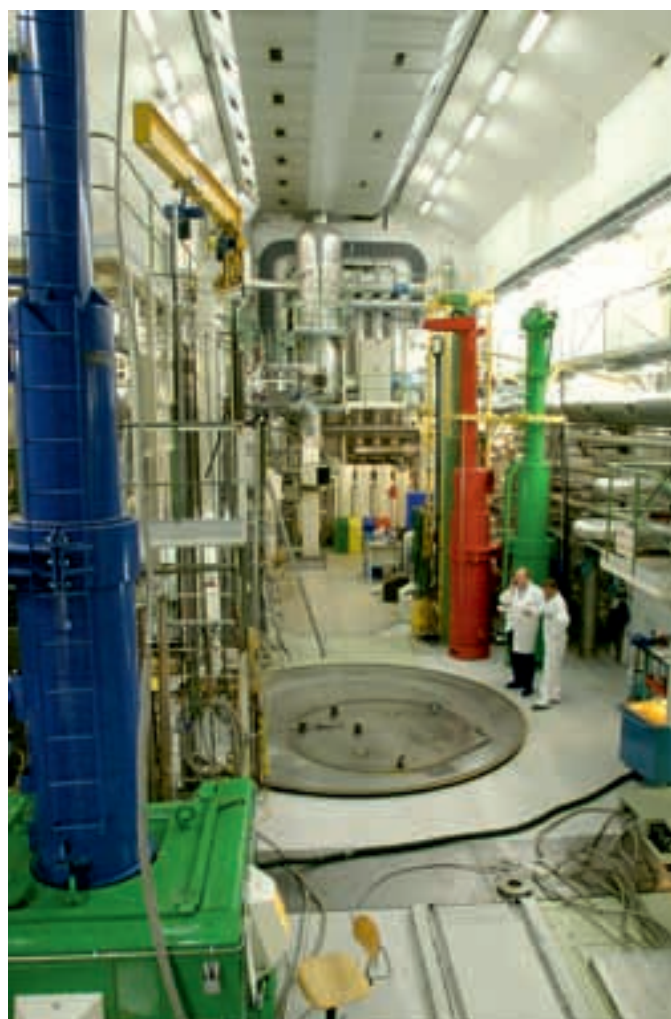
Figure 1: The Halden boiling heavy water reactor. (photo: IFE)
