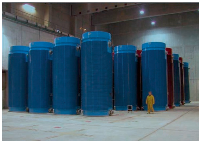
Figure 4: Storage hall with storage casks.
