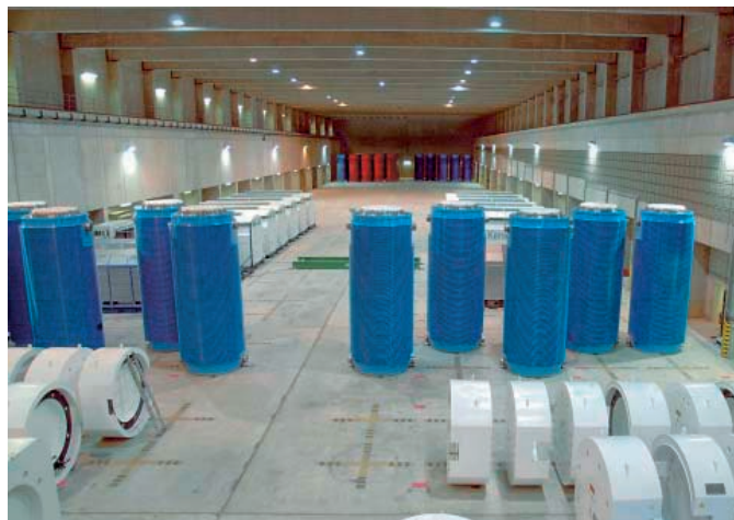
Figure 3: Storage hall with newly arrived casks and shock absorbers in the foreground.
