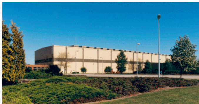
Figure 1: View of the Gorleben interim dry storage facility.
