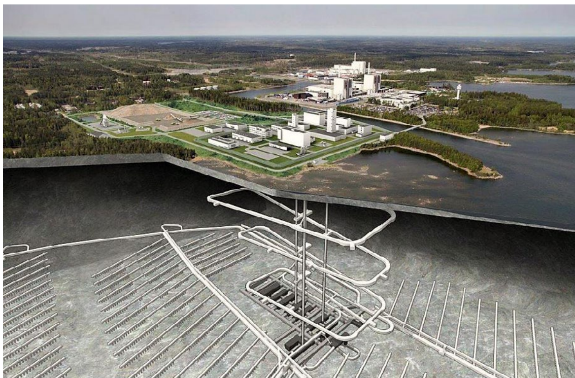
Figure 1. Design of the geological repository proposed for Sweden with its 66-kilometre of tunnels. Source: SKB.
