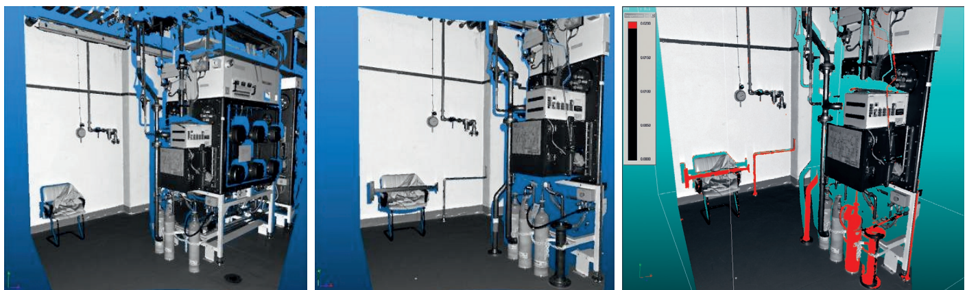
Figure 5: Reference model (left), verification scan (middle), automatically detected differences in red (right).
