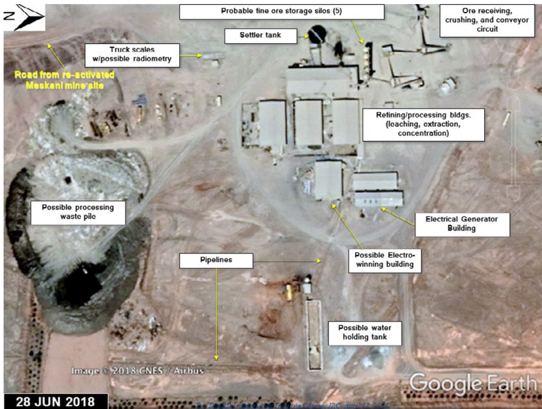
Figure 8: Mid-2018 view of the new small ore processing facility serving the newly re-activated, adjacent, Meskani mine. Labels identify the more likely roles of each part of the facility and are not meant to be definitive.
