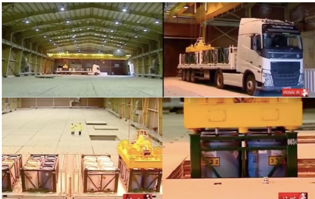
Figure 5: Interior views of the main concrete vault storage building as seen on an Iranian publicly posted video. See: https://www.youtube.com/watch?v=_bQTYpz3ylg
